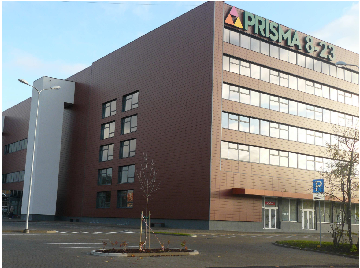
Figure 5. Trading center and Supermarket Riga, Latvia; 6000 sqm TL vertical frame system; Cladding – Creaton Tonality® clay tiles
